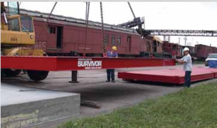
Module C is lowered into place.
