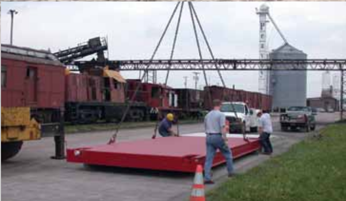
Module A is unloaded from the truck and placed on the foundation.
